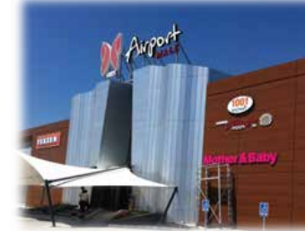
Airport Mall | Cyprus 3 x 700 kVA (Synchronized)
