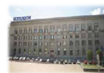
Beltelecom | Belarus 1 x 1385 kVA
