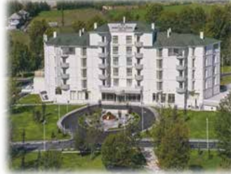
Qafqaz Yengice Thermal Hotel | Azerbaijan 2 x 1125 kVA (Synchronized)
