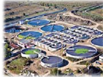
Halac Water Purification Plant | Turkmenistan 2 x 1125 kVA
