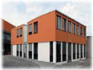
Container Production Plant Dusseldorf | Germany 1 x 400 kVA
