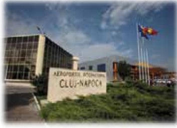
Cluj Airport | Romania 2 x 400 kVA
